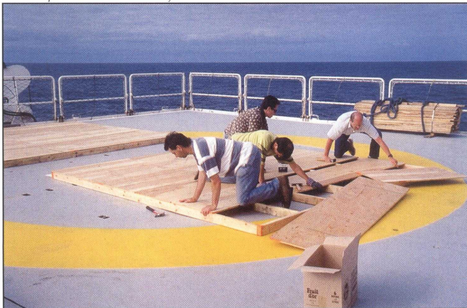
The team pre-assembled the shelter floors on the helo deck.
